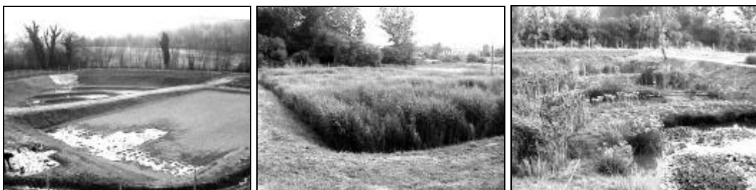
Fig. 3 – Cecchi winery treatment facility during realisation (left), SFS-h after reeds growth (middle) and well developed FWS (right)
